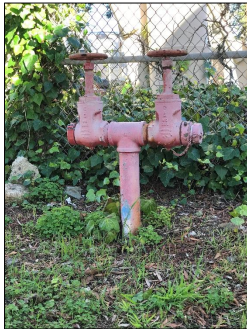
Water Tank Gated Outlets
