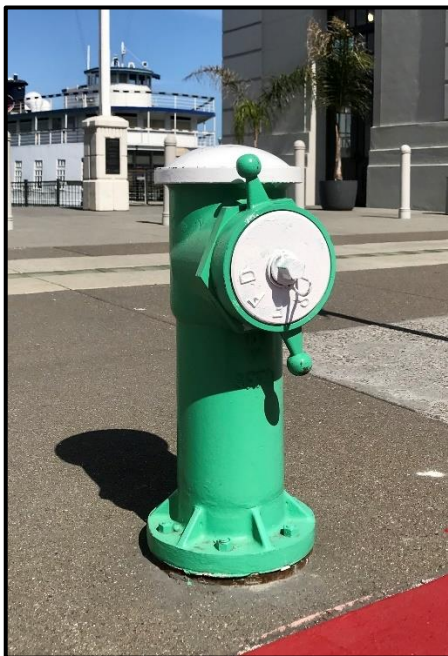
Surface Mounted Curbside Hydrant
