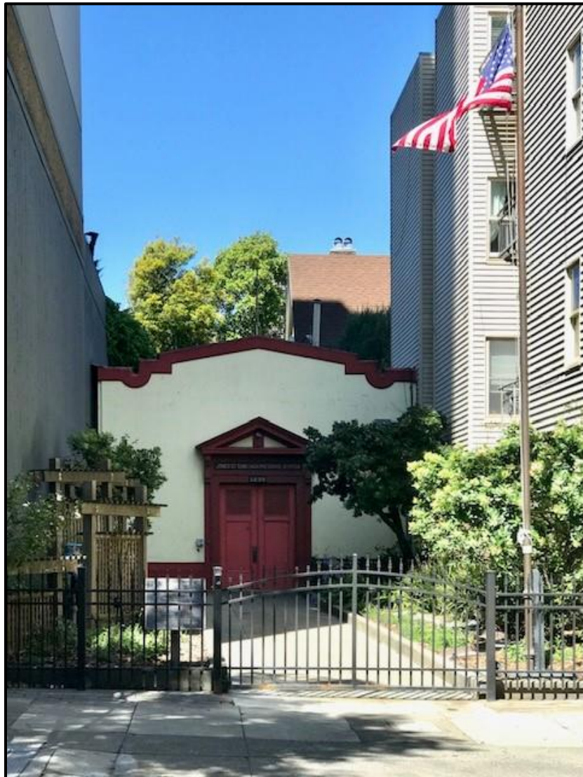
Jones Street Tank
