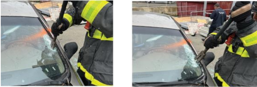
Cutting a Windshield Along the A Post with a Halligan
