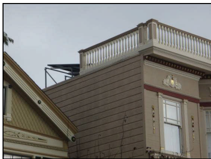
Figure 27- Elevated rack mount on flat roof in Noe Valley
