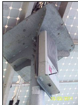
Figure 34 – Inverter installed under the PV array on Ground Mounted PV at Caesar Chavez Elementary.
