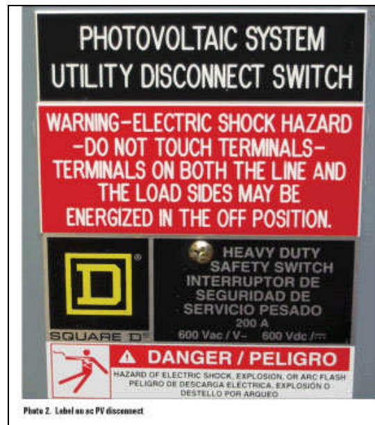
Figure 21- DC and AC power disconnect labels. Warning: “ Line ” and “ Load ” sides of any disconnect switch box could still be energized and present a shock hazard, even after the disconnect switch has been placed into the “OFF” position. This is generally the result of having dual power sources and the potential for backfeed of electrical power throughout the system
