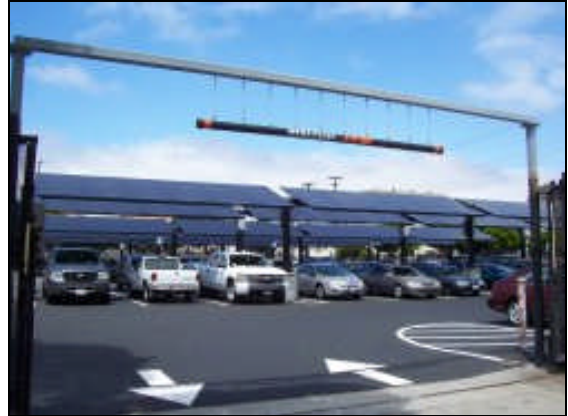
Figure 37 – PG&E Parking Structure with PV tracking system between Shotwell and Folsom at 18th street
