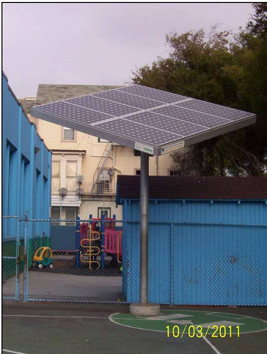
Figure 33 – Ground Mounted PV system at Caesar Chavez Elementary between 22nd and 23rd Street, Folsom and Shotwell
