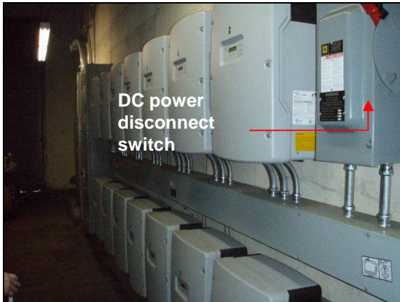
Figure 12 – Multiple System Inverters for a large commercial PV system; Cesar Chavez and 3rd Street
