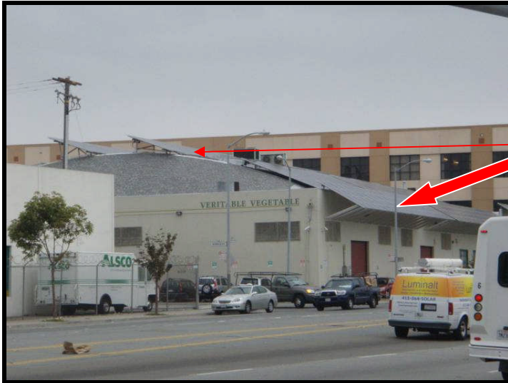
Figure 3 - Large Commercial Solar Photovoltaic (PV) system on a Type II Commercial Warehouse with a bowstring roof, Cesar Chavez and 3rd street
