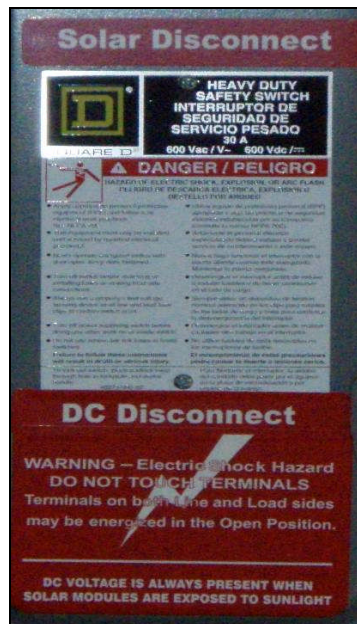
Figure 21- DC and AC power disconnect labels. Warning: “ Line ” and “ Load ” sides of any disconnect switch box could still be energized and present a shock hazard, even after the disconnect switch has been placed into the “OFF” position. This is generally the result of having dual power sources and the potential for backfeed of electrical power throughout the system
