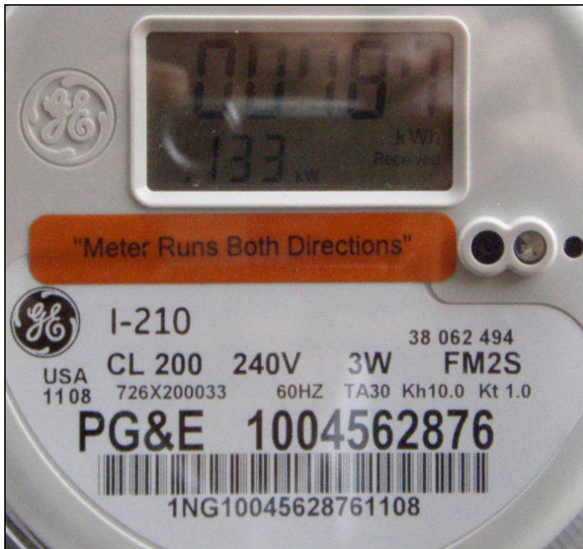
Figure 19 - Bi-directional meter labeled to indicate the presence of an alternate power source (PV). Bi-directional meters will be present on all "grid-tied" Solar PV systems.
