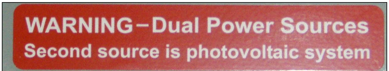
Figure 18 – Warning label on the front of a Main Electrical Service Panel (circuit breakers). The label in this instance clearly identifies that the secondary power source is solar PV.
