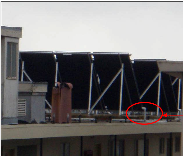
Figure 5 - Large Solar Thermal system on a 3-story Type V Multi-Unit Apartment building; 22nd and Collingwood Street, Noe Valley
