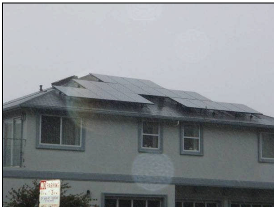
Figure 25– Roof top Residential PV system on an apartment building near Stern Grove
