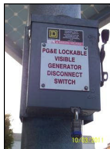
Figure 35 – Disconnect located underneath the PV array at Caesar Chavez Elementary.
