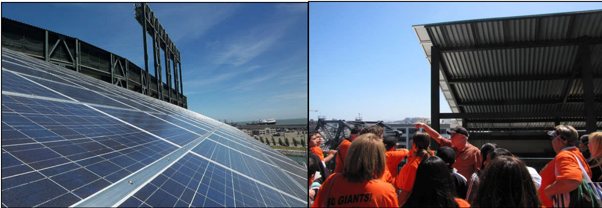
Figure 30 – Building Integrated PV system at AT&T Park. Promenade walkway cover with PV.
