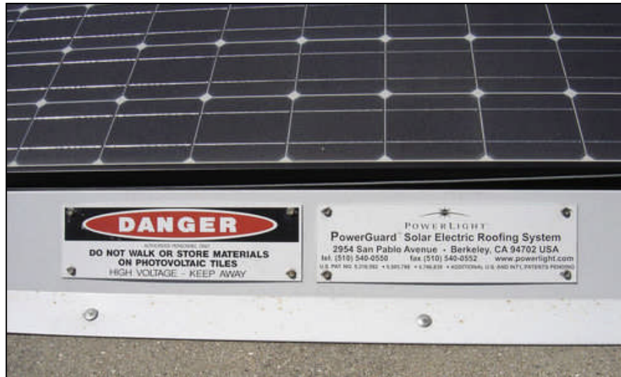
Figure 20 - Label on the side of a Solar PV module installed on the roof of the Moscone Center, provides Firefighters with a reminder of potential hazards as well as the name of the electrical contractor who installed the system.
